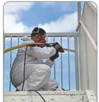
Painting & Blasting Insulation & Scaffolding
